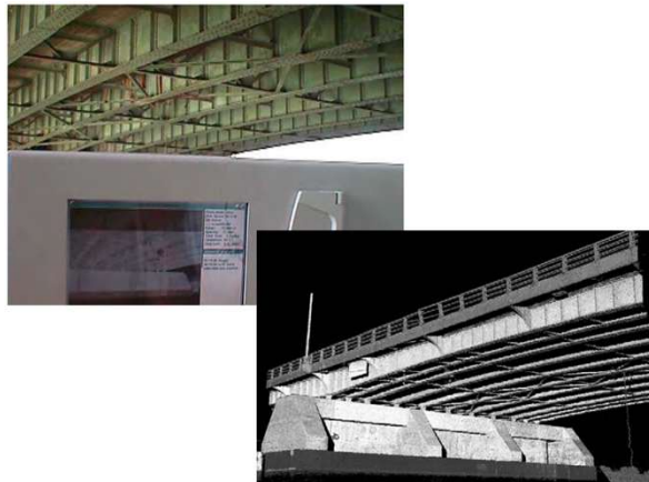
Figure 9: Optech LIDAR scanner and resultant image of underside of Kennedy Bridge.
